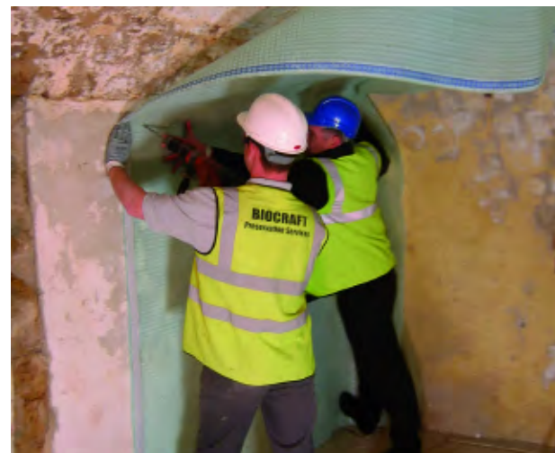
Installing Platon Multi
